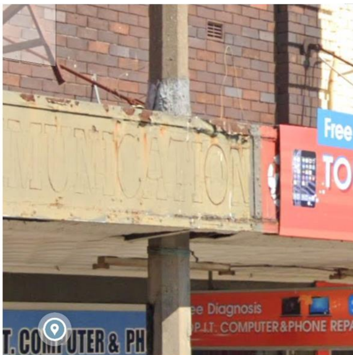
The street awning is inappropriately constructed around the streetlight column. Source: Google Maps Street View.
